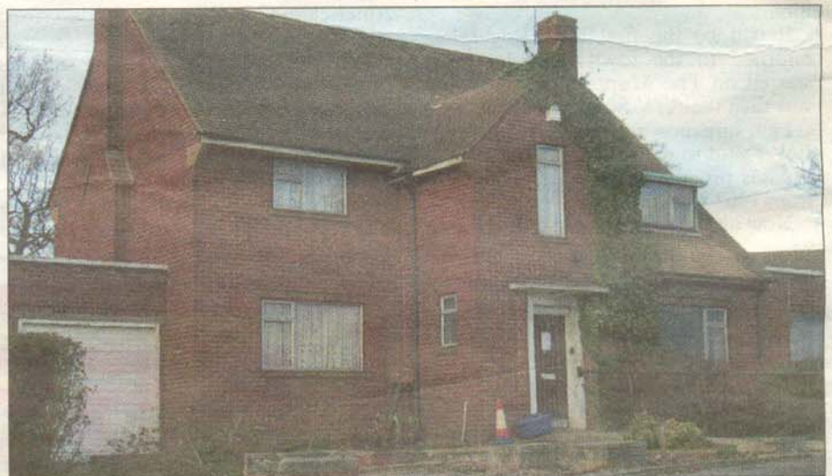
'Inadequate': the former Grove Road site where the practice spent 53 years
